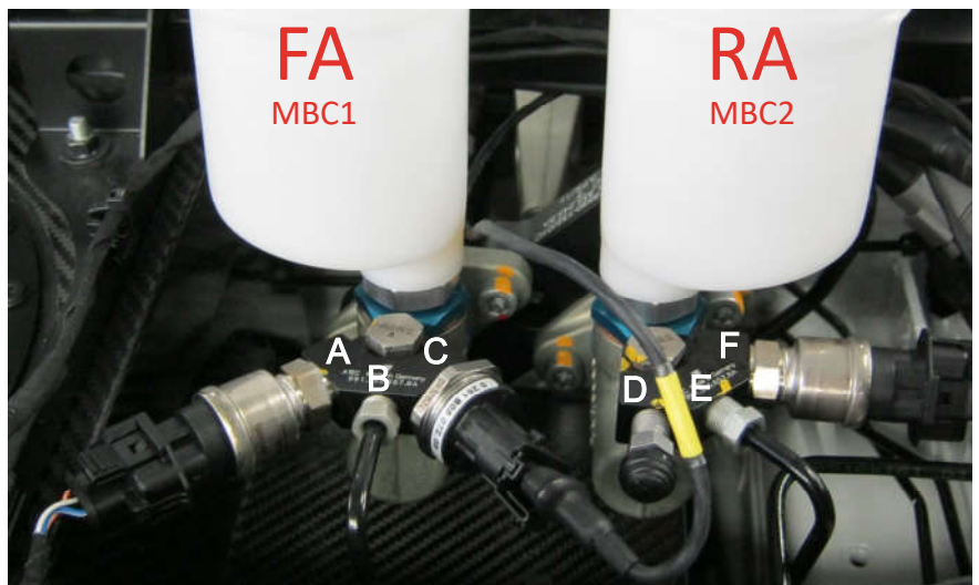
Step 7: Shows the already rebuilt brake lines and pressure sensors
